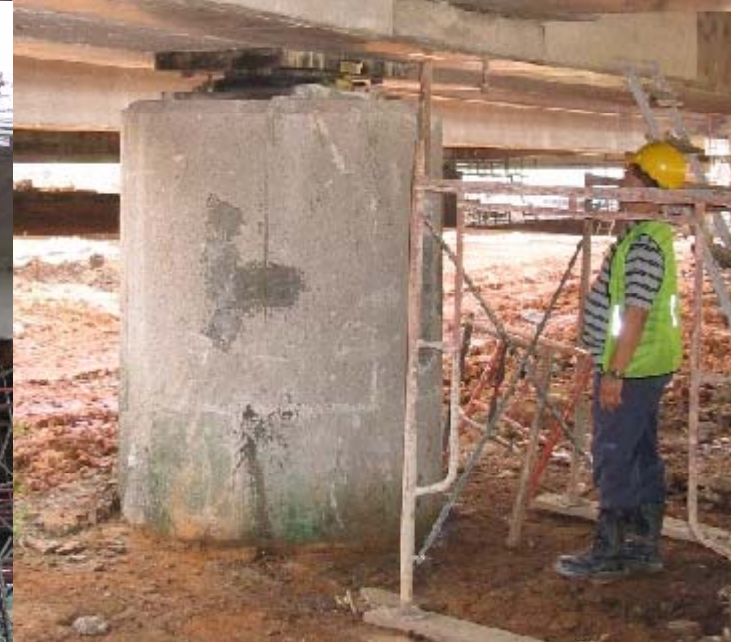
Photo Source: SysEng (S) Pte Ltd
